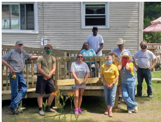
Jackson County disAbility Connections building a ramp for a community member
